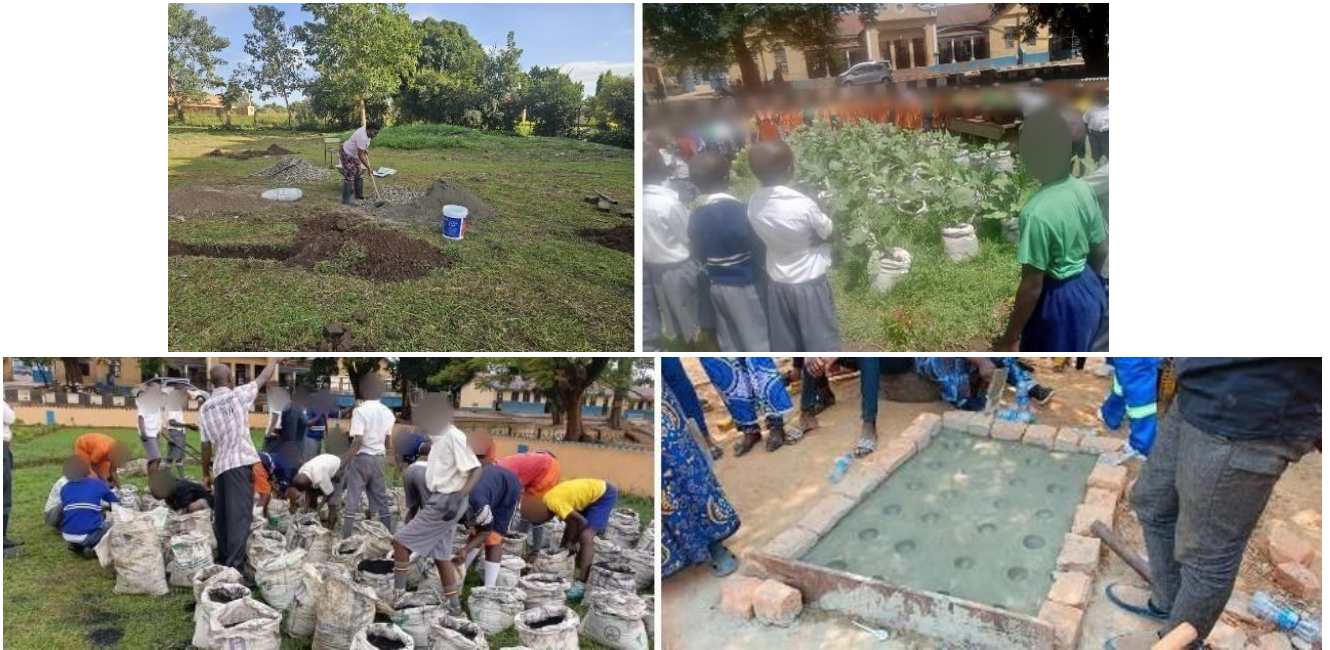
Figure 5: Construction of low-cost learning centres with learner and community participation under Code 7.
